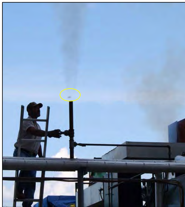
Photo #4: Yellow circle identifies the mach line during a steam blow
